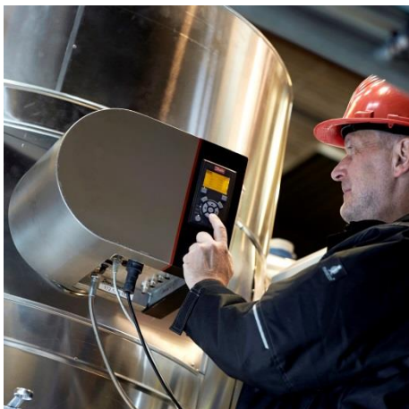
Illustration 3: The Sensor Unit Mounted on the Exhaust Pipe
