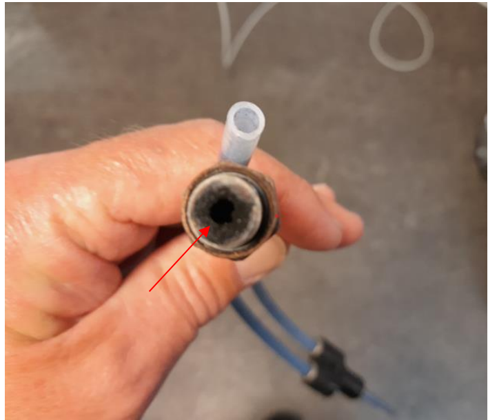
Air hose clogged with soot
