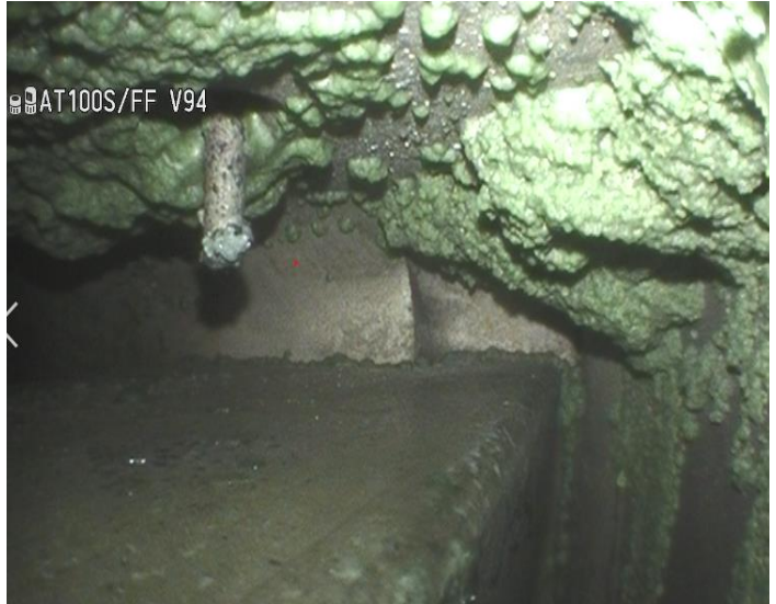
Soot deposit inside the probe
